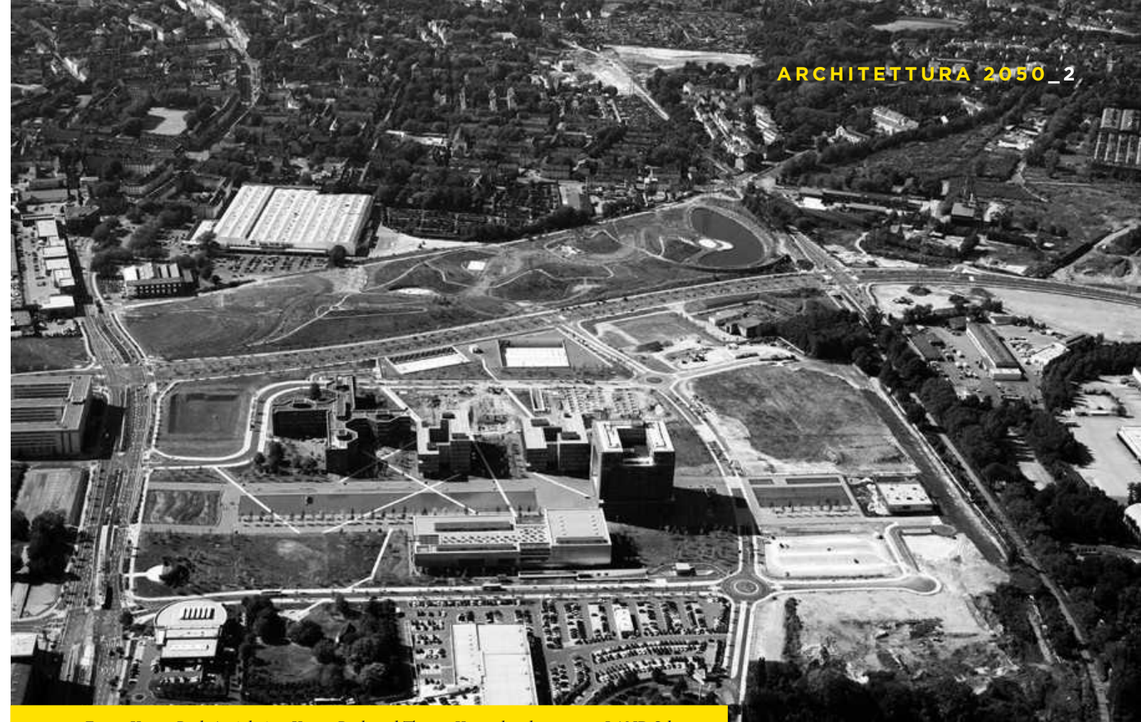
Essen, Krupp Park Aerial view Krupp Park and ThyssenKrupp headquarters ©LAND Srl
