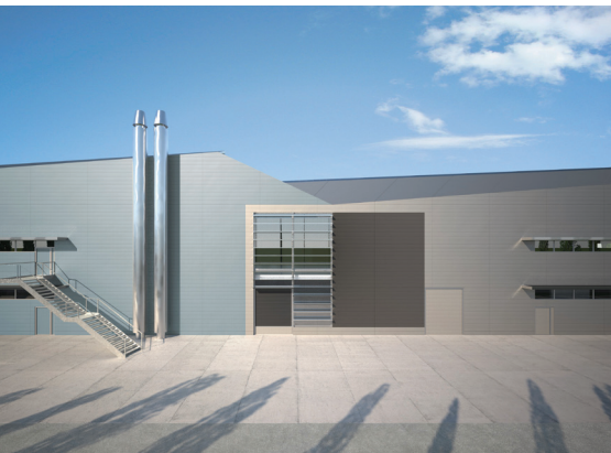
Petronas R&T Centre, Santena (TO) © 967 Architetti Associati
