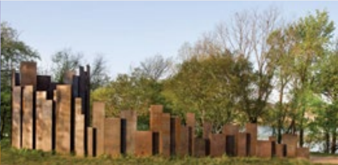
Trail Restroom - Arch. Mirò Rivera
