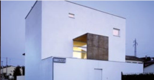
NEW ARCHITECTURES PRIZE: Casa Cavazzana - Enrico Franco
